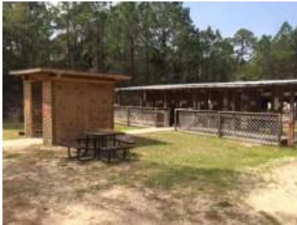
Figure 2. Range A Entry Control Point
