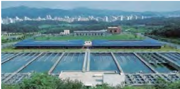
■ Seongnam Water Treatment Plant
